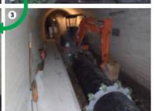
③ Loading of Pipes with a Backhoe
