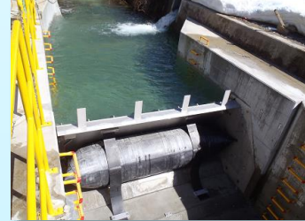
Water Intake Weir (Lodging Weir)
