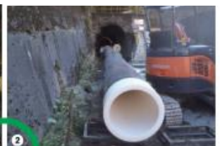
② Forming Long Pipes by Welding
