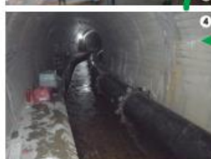
④ Pipe Loading Completed
