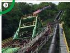
③ Penstock Installation Preparation
