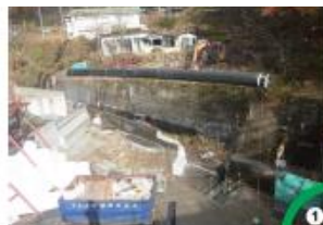
① Delivery of a Series of 10m-long Pipes
