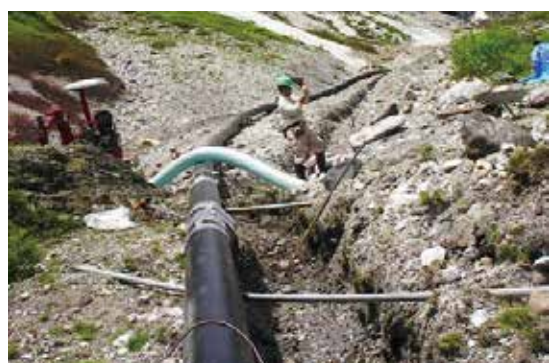
●配管布設状況●
